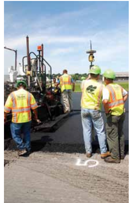
Topcon dealer Jim Cleary checks the grade with the GR3 Survey Rover.
